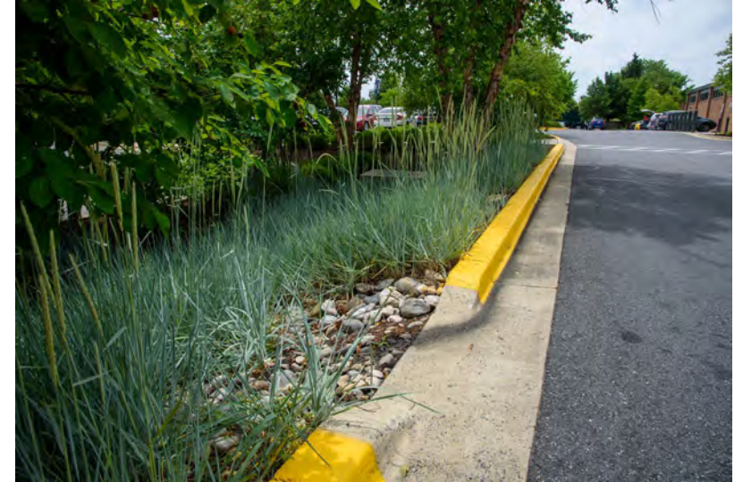
Curb cut to rain garden, bioswale Source: Prince George's County Planning Department
