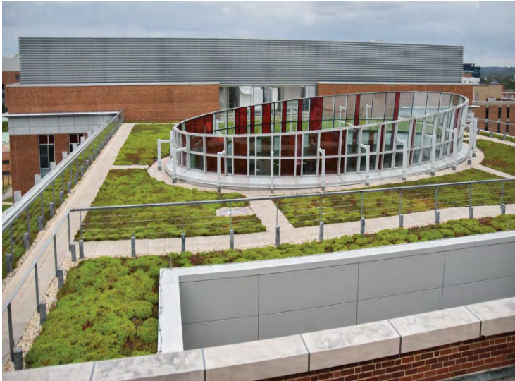
Green Roof at University of Maryland, College Park Source: Joe Ryan/The Diamondback Newspaper
