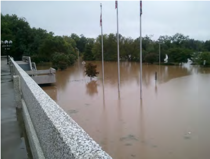
2011 Flood, Central Administration Building (CAB) Source: Prince George's County Planning Department
